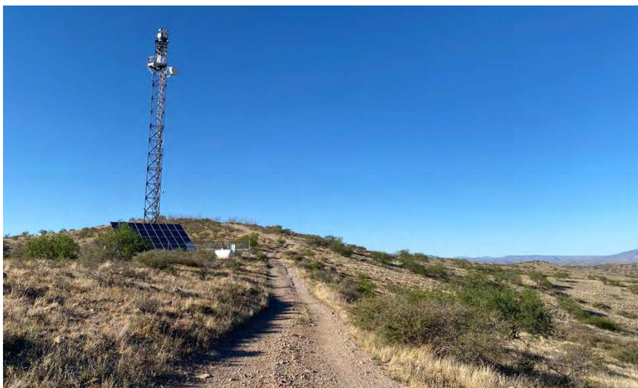
Photo 2. Elbit Systems AI surveillance tower, Arizona.
