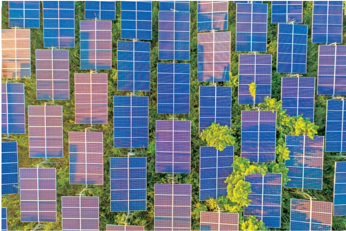
Solar panels aerial view.
