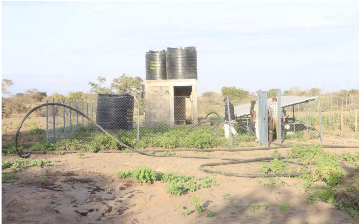
CAN-Tanzania project, to provide water for irrigation to the people in Kilimambogo, Tanzania. PHOTO/ PSA
